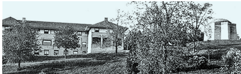
ALPHA DELTA PHI CHAPTER HOUSE AT CORNELL UNIVERSITY, ITHACA, NEW YORK. GEORGE R. DEAN, ARCHITECT, CHICAGO, IS DESIGNED TO STAND ON A POINT OF GROUND OVERLOOKING THE CITY. THE LARGE PLATE-GLASS WINDOWS IN LIVING-ROOM LOOK UP AND DOWN THE VALLEY. THE TWELVE-SIDED PORCH HAS WINDOWS THAT SLIDE UP INTO THE WALL OR MAY BE PULLED DOWN IN WINTER, INCREASING THE LIVING-ROOM SPACE. THE BUILDING WILL BE OF BRICK AND PLASTER WITH STONE BASEMENT AND TILE ROOF. THE LODGE STANDS ABOUT TWENTY FEET HIGHER ON THE GROUND THAN THE HOUSE, THE ENTRANCE BEING APPROACHED BY A FLIGHT OF STEPS
