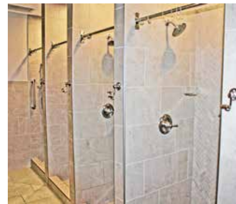
BELOW: Four large, stone-tiled, individually-lit shower stalls with durable stainless steel fittings are conveniently installed on each dormitory floor.
